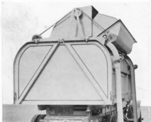
Bucket entering enclosure about to assume its dumping angle of 45 degrees
