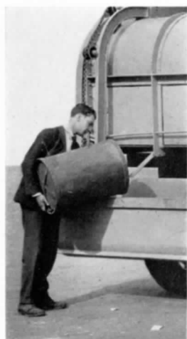
Easily loaded. Only 30 in. lift above curb required.
