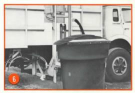
This unit is picking up a 300-gallon container, ideal size for apartments, alley collection for close-spaced homes, light commercial use.
