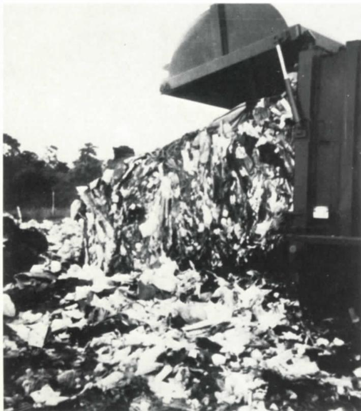
Xtra High Density packing shows up in a solid payload . . . like toothpaste coming out of a tube. This Xtra compaction is the result of the Dempster engineered tailgate, designed to rotate refuse as the compaction cycle takes place. As it rotates, refuse is compacted over and over by a specially shaped packer head, until every corner of the body is filled. The new Dempster Roto-Dor tailgate really works.
