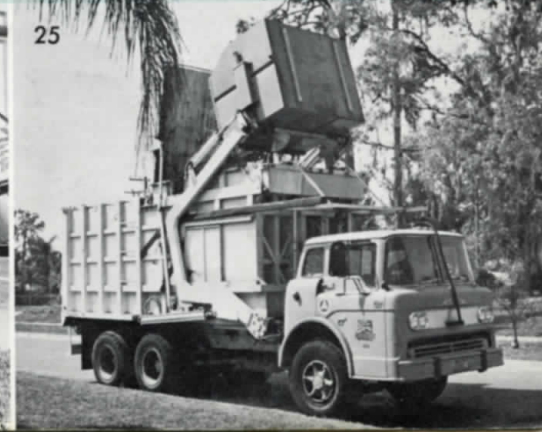
■ Photo 25. The trimmings are transferred to the compaction chamber where they are reduced to a fraction of their former volume.
