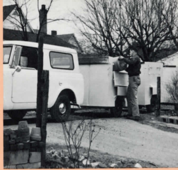
ALLEY PICKUP Because of its mobility, the container train is well suited to alley pickup. Here a member of the loading crew empties refuse into a train container in a narrow alley.
