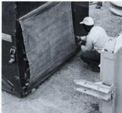
Tight fitting canvas cover is fastened to prevent spillage while container is enroute to the disposal site.
