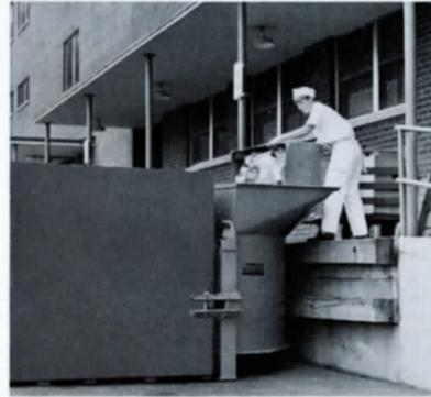
PowerMite can be set flush against a dock. No special dock board is needed. Loading hopper is optional.
