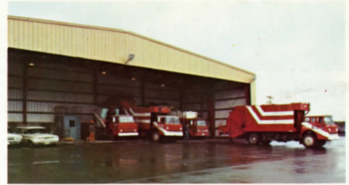
Two Transfer Packers and two Push Pits provide space for several collection vehicles to unload at one time.
