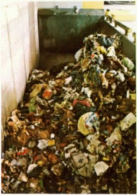
Push Pit provides temporary refuse storage.
