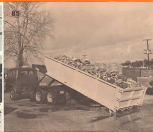
Gigantic load of brick is picked up in seconds. Ideal for wrecking work.
