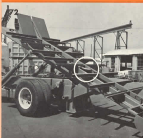
Bail cylinder pulls base up on tipping frame which is then lowered.
