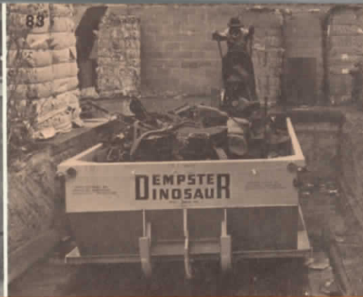
Low construction container is ideal for use with scrap metal storage.
