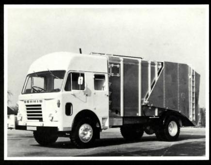
"Automatic loading compression type refuse-collector" (With tipping discharge)
