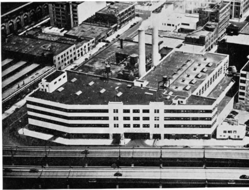
West 56th Street Incinerator, which also houses a garage.
