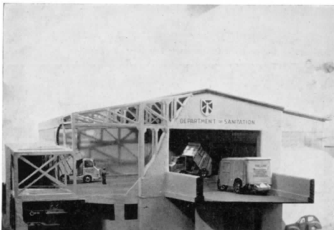
Scale model of enclosed waterfront disposal station. Trucks enter from ramp. Note truck (left) dumping into barge anchored underneath.
