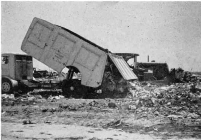
Refuse is dumped. Bulldozer pushes it over bank.
