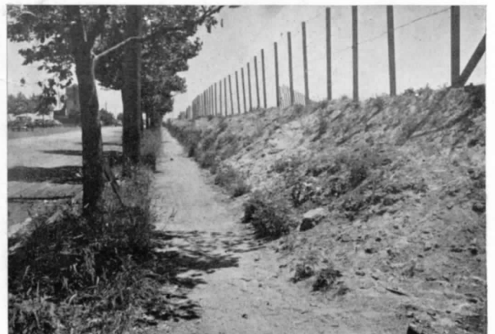
Below: Drift fence erected at start of operation.
