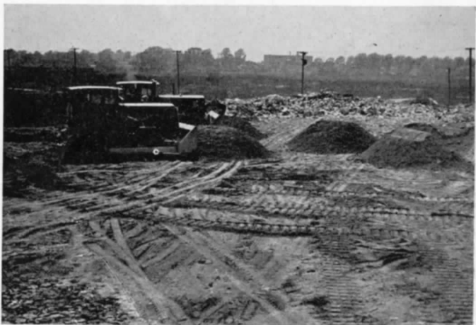
Bulldozers spread sandy cover and compact deposited material.
