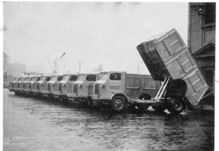
Some of new-box type trucks. Plans are under way to improve these and earlier models by adding a compactor device.
