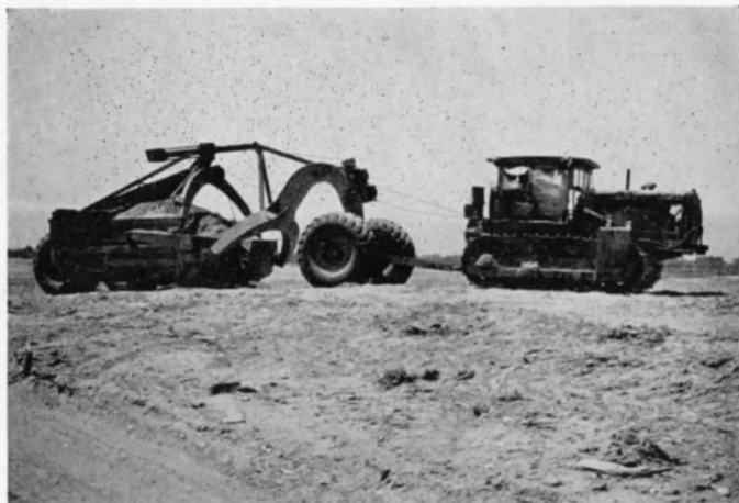
Transporting clean covering fill to active bank of landfill.
