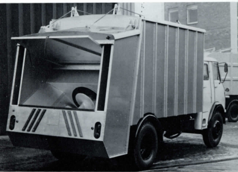
The "Musketeer" Refuse Collector, with the refuse packing screw
