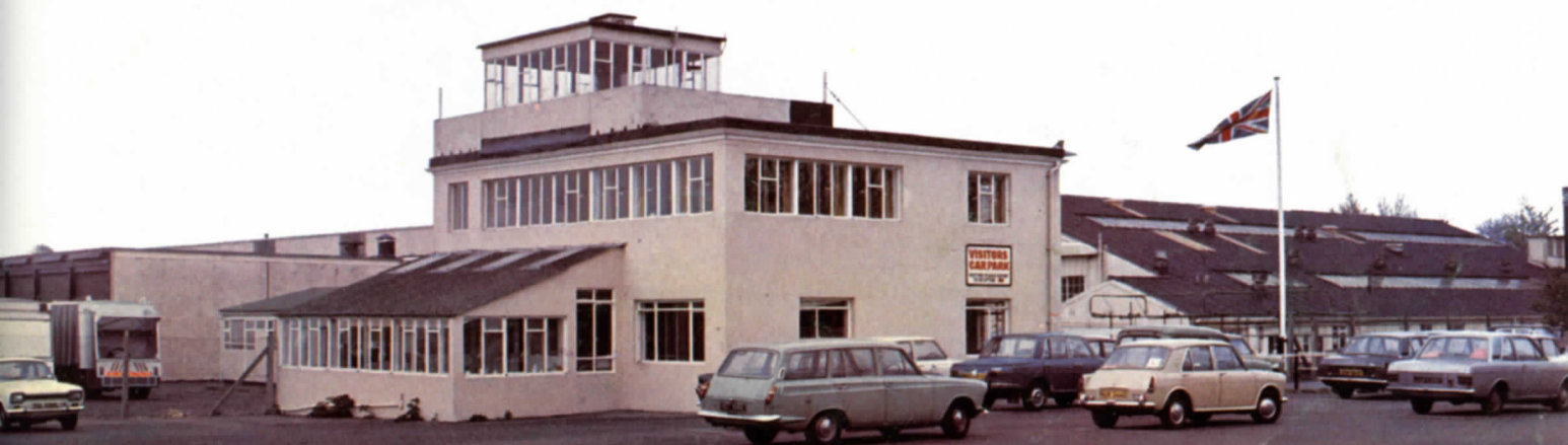
View of Glover main office and factory at Hamble, Hampshire.
