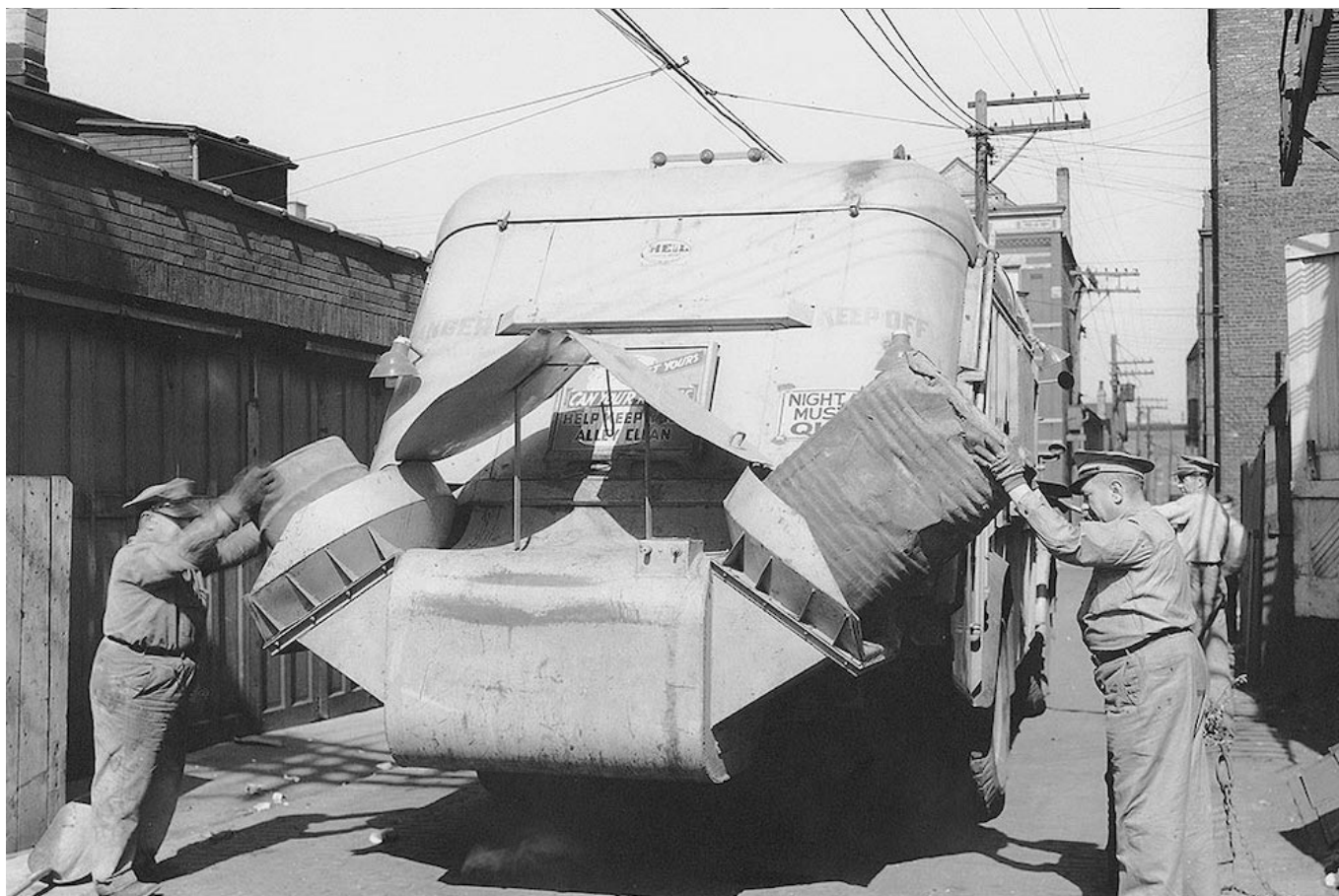
Dual openings on the Heil Conveyor sped the loading process, and kept moving flights away from crew and trash barrels.
