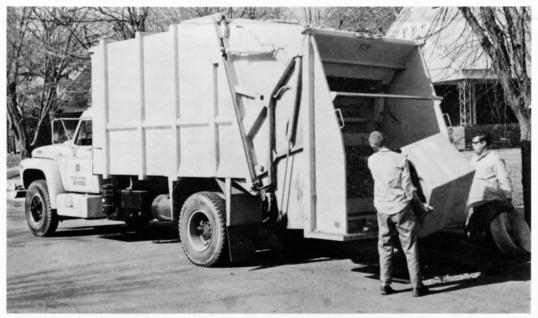
ON THE FIRING LINE: Hobbs-Pak rear-loading refuse packer brings simplified engineering, balanced design and maximum safety to the
