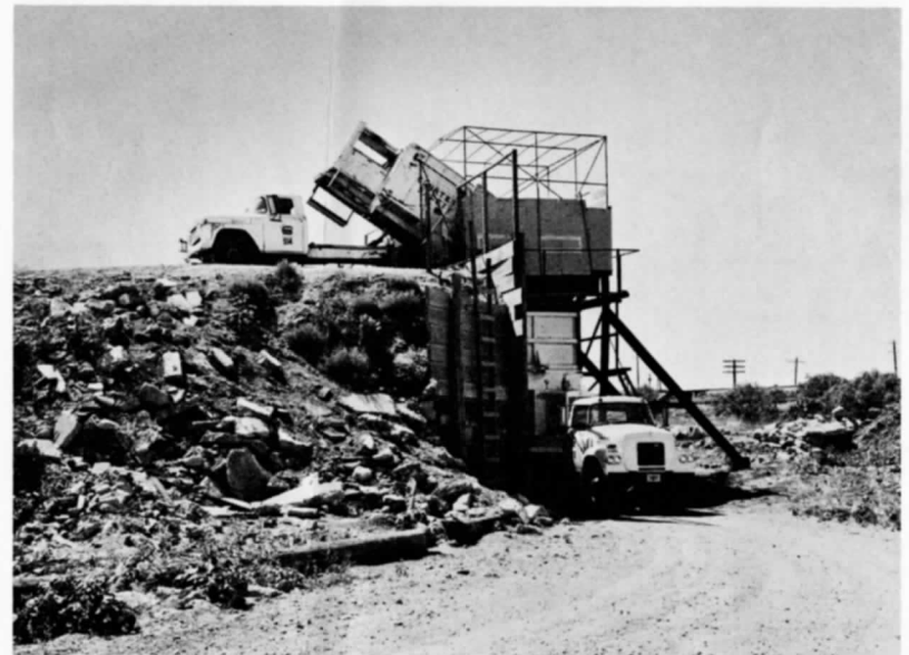
Abilene's transfer station shows dirt fill ramp construction. Shown in receiving position is one of city's two 42-yard Hobbs HYD-PAK transfer trailers.
