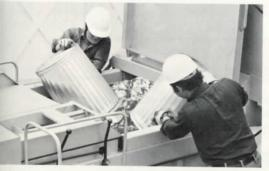
ONE MAN OR TWO MAN LOAD-ING: The EVO hopper provides low-level "downward" loading . . . . just one or two steps from curbside. The compactor plate hydraulically compresses material into the 8 cu. yd. body with very high density. Crewmen continue to load during all phases of the compaction cycle. Compaction controls are at both sides of hopper.
