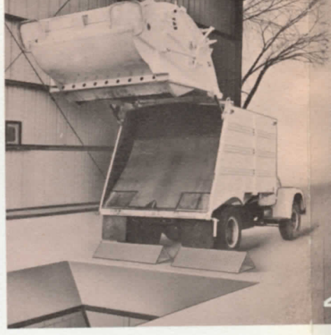
4. Top-side view of LEACH collection unit dumping of trailer on lower level showing ordinary operation.
