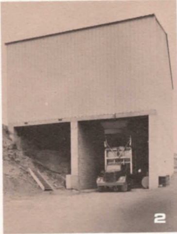
1. Front view of Hopper and Power Compaction unit. 2. Compaction Trailer in position to receive refuse from above level. Note: In this particular installation, low cost, bi-level steel-and-concrete block structure,
