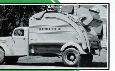
Along its route, the contents are carried in the permanently closed body, safely screened from the gaze of passersby and from the shifting breezes. Once the bucket has deposited its contents inside the body, no passerby is ever offended by the unsightly appearance of a load of refuse, never is he subjected to the unsavory odors that can be given off by open trucks on a summer day.
