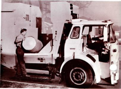
Refuse hopper directly behind cab features low pitch in height and continuous cycling, for one man drive and pitch.
