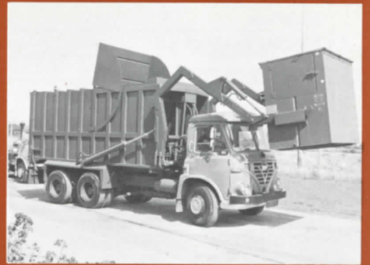
The anti-scatter guard is opened and the lifting sequence commenced.
