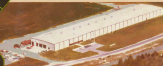
Duffield, Virginia Plant
