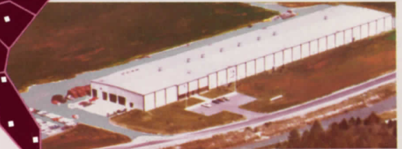
Duffield, Virginia Plant
