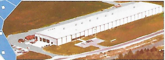
Duffield, Virginia Plant
