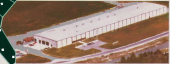
Duffield, Virginia Plant
