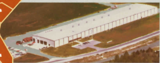
Duffield, Virginia Plant
