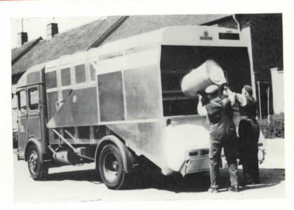
HYGIENE The large-capacity hopper is well enclosed, thus reducing dust emission to a minimum, but for those Authorities that demand an even higher standard, the SD patented compressed-air shutters can be fitted which completely seal the rear of the hopper.
