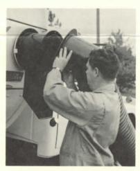
The long, heavy duty, steel reinforced vacuum hose provides excellent control and wide range of movement for the operator. The hose can be snapped on or off in a matter of seconds. Simply replace the hose with the vacuum face plate and your Tecorp unit is ready for conventional refuse collection.
