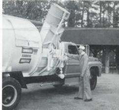
The Trux-Tilt Hydraulic Lift is optional equipment on all sizes of Truxmore refuse bodies. A simple locking device permits the operator to attach a 55 gallon drum or wheeled disposal container to the lift, dump it, and return it to the ground in less than ten seconds. Between
