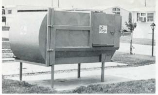
As a stationary packer, the PUP is placed at a restaurant, super market, mobile home village or any refuse generation site and operated with an electrical power unit. A whole fleet of PUPS can be serviced with only one pickup truck.
