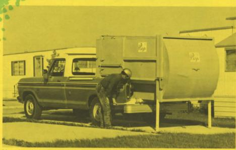
Need to use the pickup without the PUP? Just disconnect the hydraulic quick couplings, winch the PUP off on its legs and the truck is free for any purpose. Takes less than five minutes. Hoses automatically disconnect from PUP should your operator forget to uncouple them.
