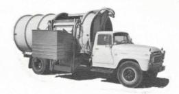
Operation of lever begins hydraulic action and container is carried to emptying position.
